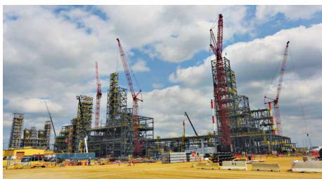
The PE1 Expansion Project has passed the 60% construction complete milestone.
